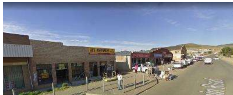
Figure 48: General view of Main Road, EmaXesibeni.
