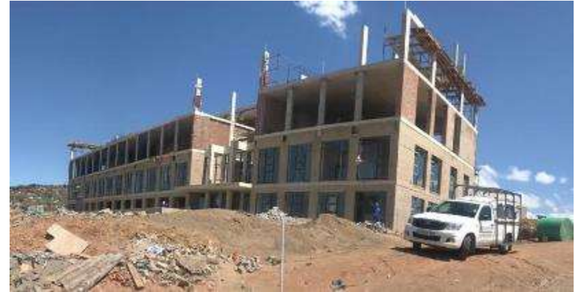
Figure 52: New Municipal Offices currently under construction in KwaBhaca.
