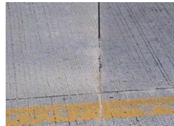
Concrete (Rigid) Road
