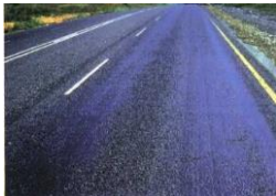
Flexible (Tar) Road
