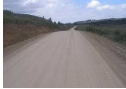
Earth (In Situ) Road
