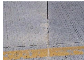
Concrete (Rigid) Road
