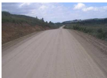
Earth (Insitu) Road
