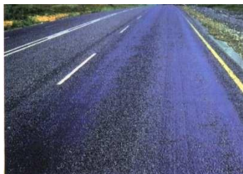
Flexible (Tar) Road
